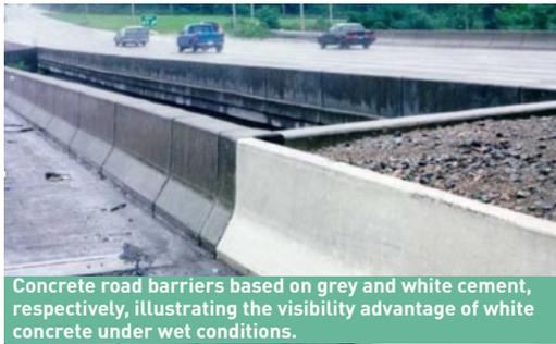
Concrete road barriers based on grey and white cement, respectively, illustrating the visibility advantage of white concrete under wet conditions.
