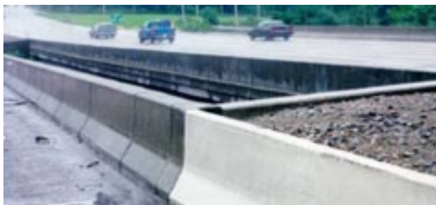
Fig. 5: Concrete road barriers made using grey and white cement, respectively, illustrating the improved visibility of white concrete under wet conditions
