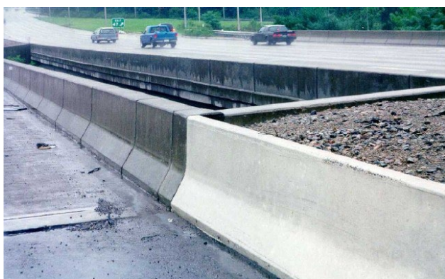
Fig. 7: Concrete road barriers made using grey and white cement, respectively, illustrating the improved visibility of white concrete under wet conditions.
