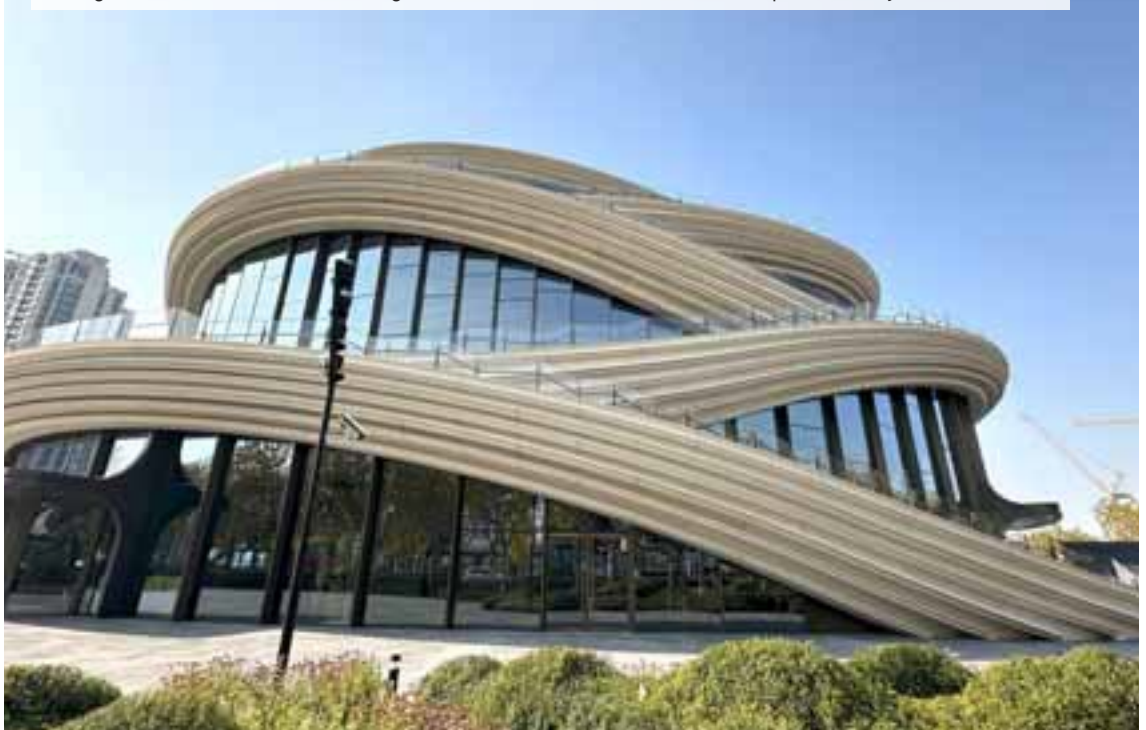
Shanghai West Bund Orbit-Aalborg White based GRC facade elements produced by Zhuohai Shantai
