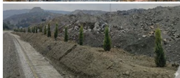
Rehabilitation in Izmir
