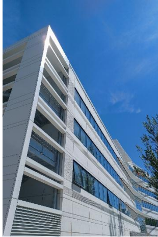
1. Precast concrete façade (D-Carb Lower Carbon White Cement)
