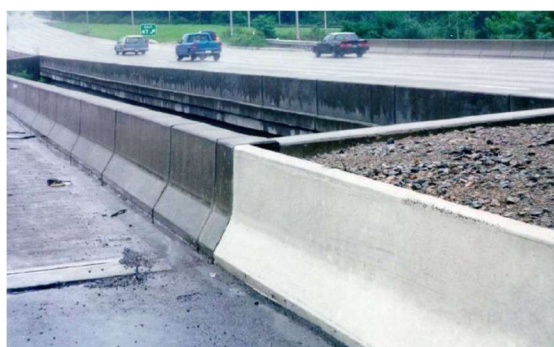
Left: Concrete road barriers based on grey and white cement, respectively, illustrating the visibility advantage of white concrete under wet conditions.
