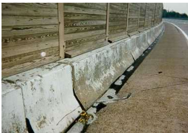
Fig. 8: Grey concrete road barriers painted white. Illustrates the safety hazard and additional costs needed for repainting the road barriers.
