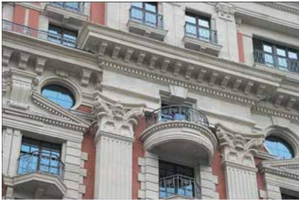
The classical style of the precast ArchiStone® cast stone elements based on Aalborg White® cement on the first six floors completed the strong and solid image of the building. The highly refined decorative concrete elements, coffered ceiling balconies, rusticated corners look amazing on the exterior of this international luxury hotel — The Ritz-Carlton.
