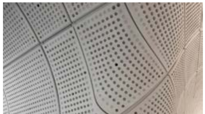
These geometrically complex concrete elements in the Crossrail Farringdon Station, London, England, demonstrate the strong potential of UHPC mixtures for architectural precast concrete (photo courtesy of mbX, Bergen op Zoom, the Netherlands)
