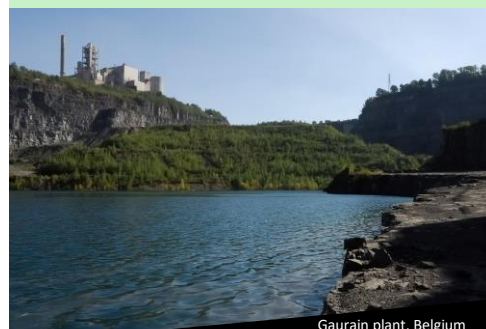
Gaurain plant, Belgium
