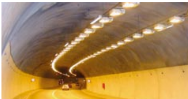
Fig. 4: Application of white cement-based panels reduces need for lighting in an underground tunnel
