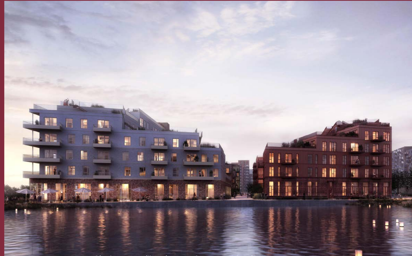
▲ FUTURECEM was used in the UN 17 Village in Copenhagen, Ready-Mix Concrete supplied by Unicon and managed by the construction company CG Jensen. The project designed by Sweco Architects and design layout by Lendager Group
